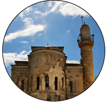
FİSANDON MOSQUE – CHURCH
